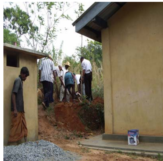
Fig. 7 Installation of lightning protection towers
