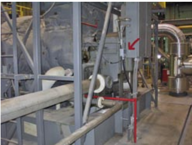
The Vaisala HUMICAP ® Moisture and Temperature Transmitter for Oil HMP228 is inserted directly into the line with ball valve assembly. The unit is installed in a bearing return oil drain adjacent to the high pressure end turbine packing.
