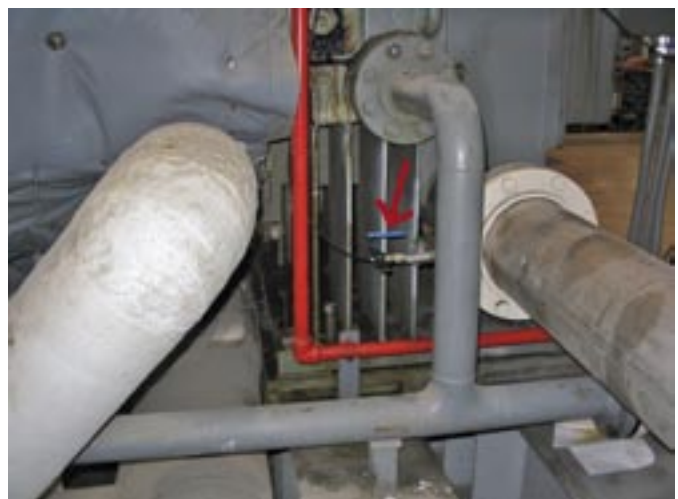
The Vaisala HUMICAP ® Moisture and Temperature Transmitter for Oil HMP228 is inserted directly into the line with ball valve assembly. The unit is installed in a bearing return oil drain adjacent to the high pressure end turbine packing.
